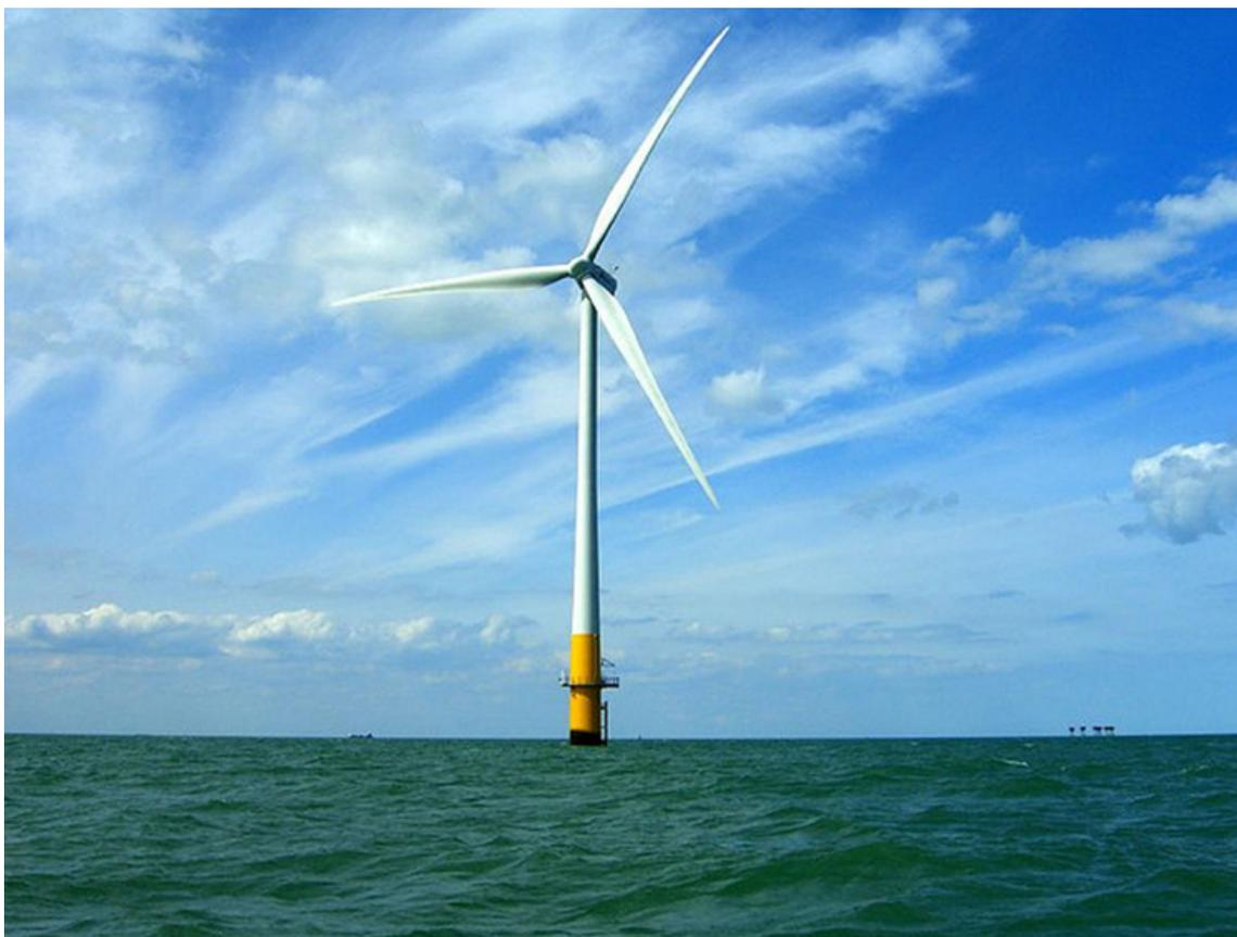
**Figure 1:** This wind turbine in the Thames Estuary in the UK is an example of induction at work. Wind pushes the blades of the turbine, spinning a shaft attached to magnets. The magnets spin around a conductive coil, inducing an electric current in the coil, and eventually feeding the electrical grid. (credit: phault, Flickr)
